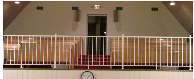
The other very visible safety feature is a new railing at the front of the balcony. There is a clear plexiglass portion at each end of the railing as well so that there are no gaps through which anyone might fall. The previous railing was quite low so this will provide an extra measure of safety.
